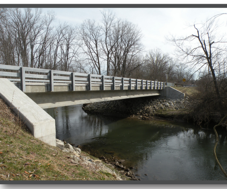
Moorefield Road Bridge No. 447
